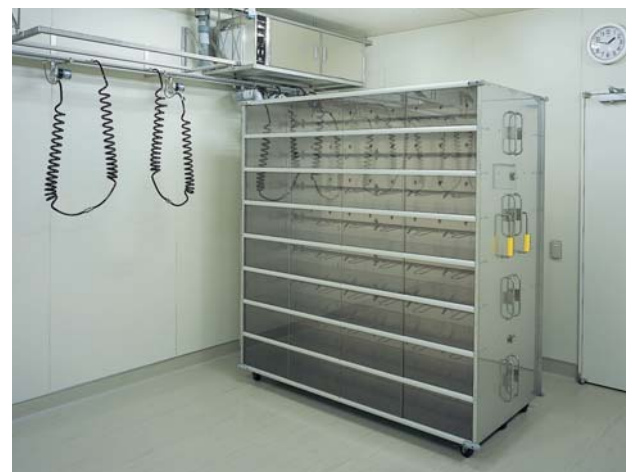
Example: Installation of custom-designed Safety Rack
